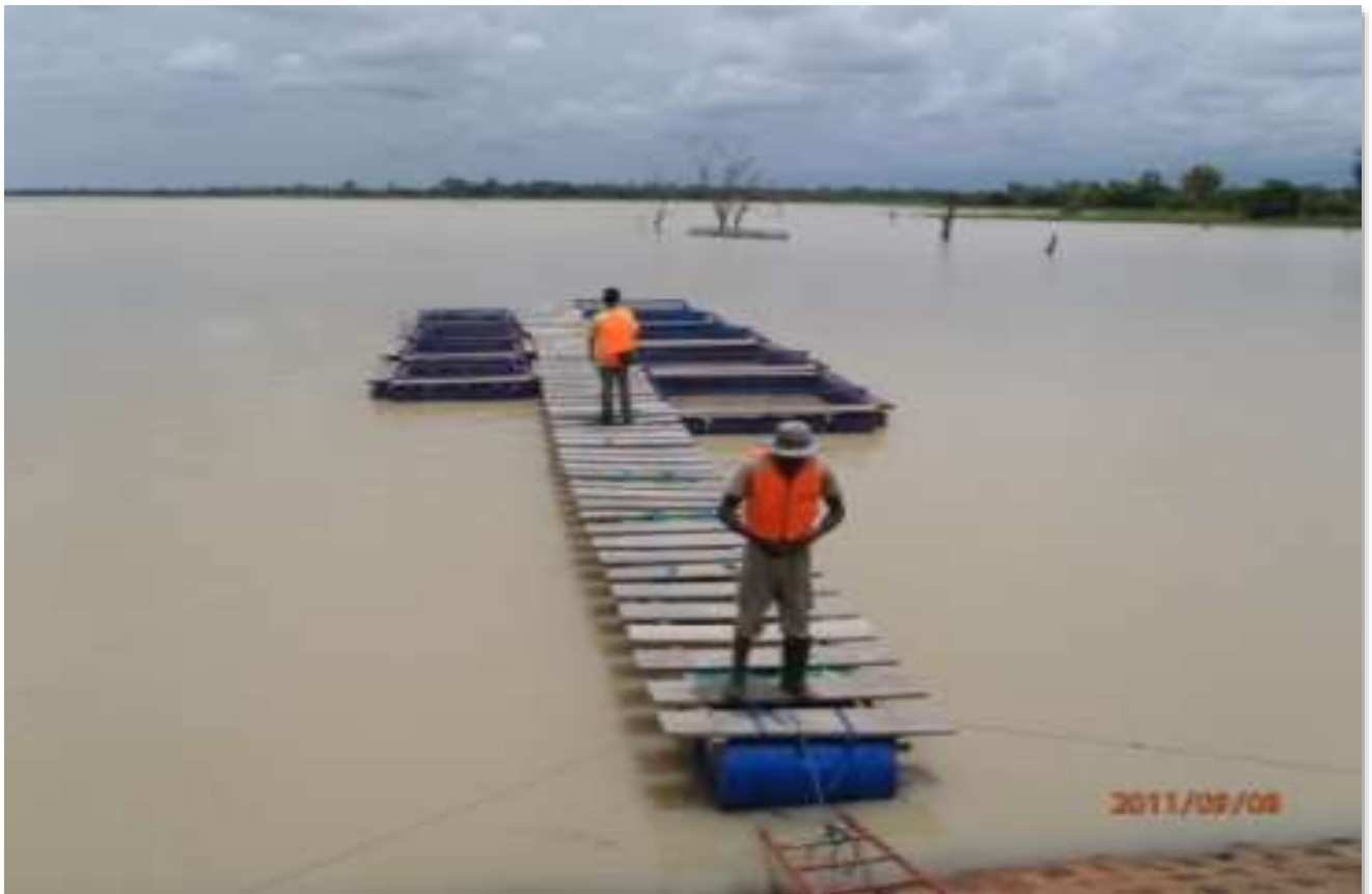
Photo 13: cages flottantes installées
