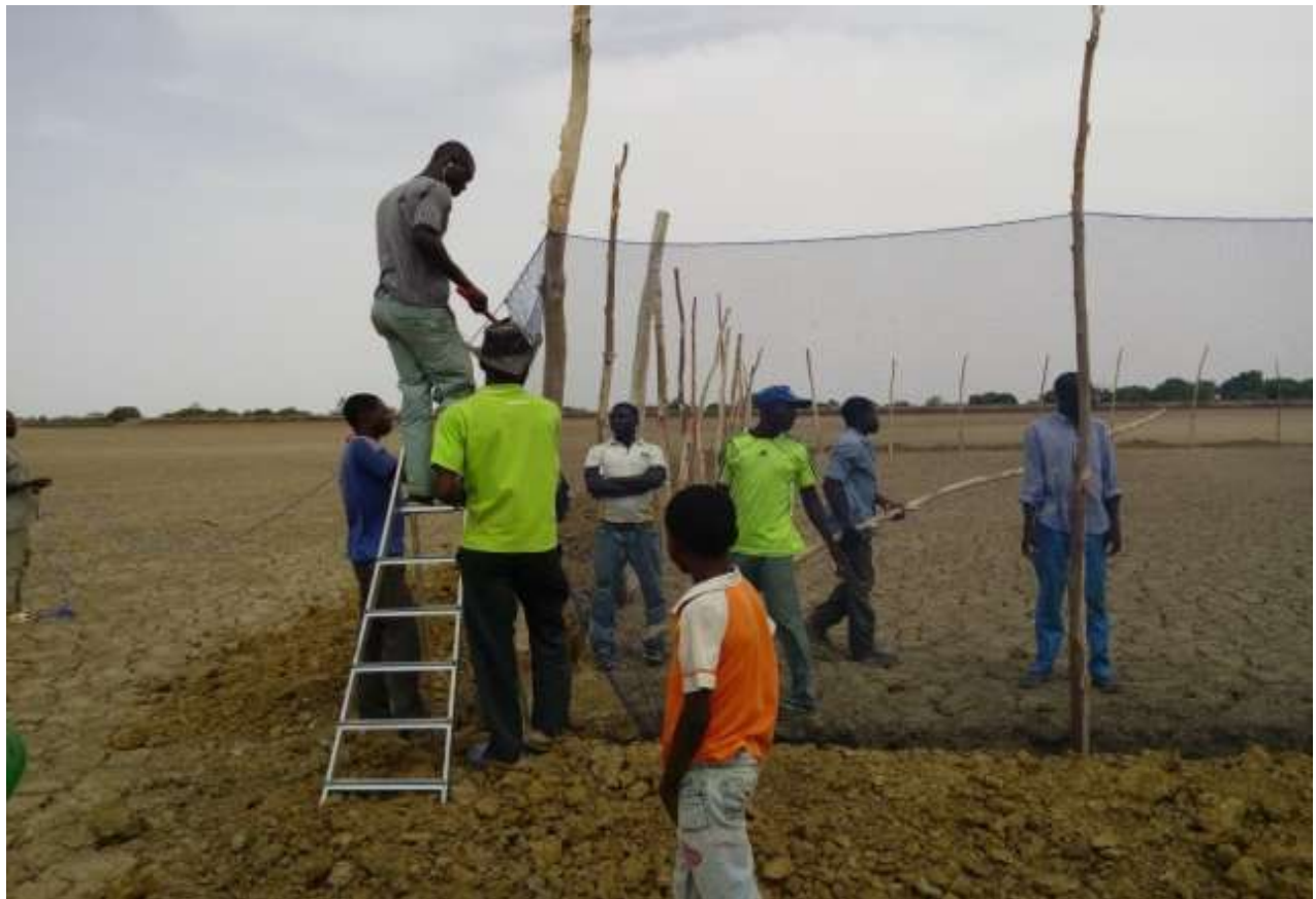
Photo 6: Enclos piscicole en construction
