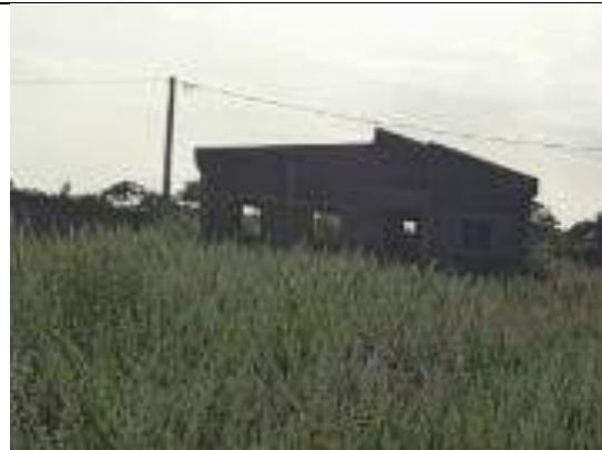
Photo 6: Infrastructure en finition
