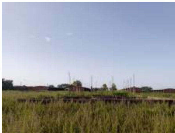
Photo 5: Infrastructure non achevée
